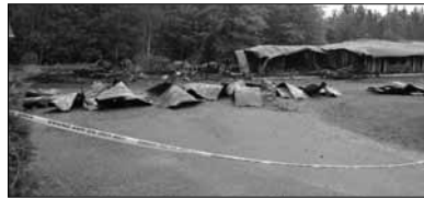
A major portion of the Blue Moon Motel in St. Andrews was destroyed by fire in the early morning hours of Saturday morning. Here, the metal roof lays curled in the parking lot Saturday.
